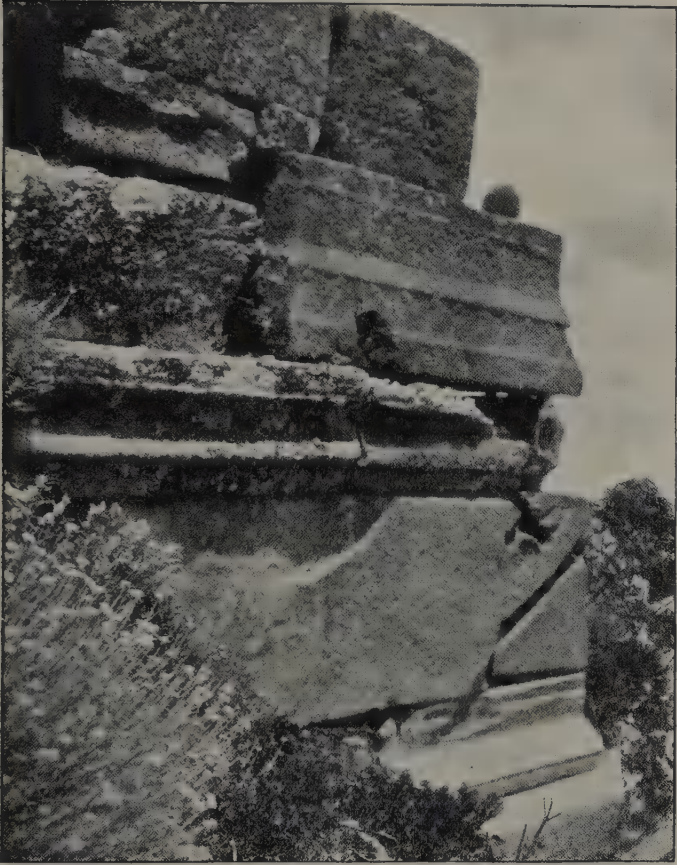
FIG. 282.—Kurshundju, monastery wall built of re-used stones.
